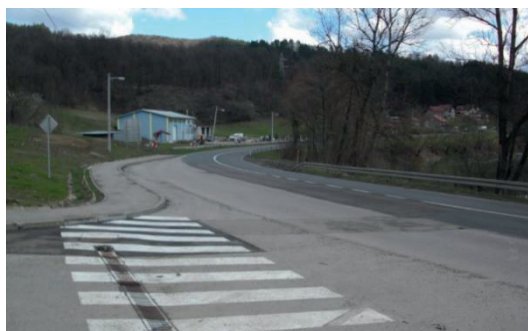
Picture 2. Condition on the subject spot from 2011 (Google earth, 25 October 2016)
