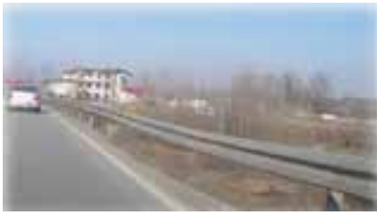
Figure 5. Poor maintenance (M16.1)
