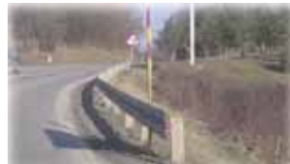
Figure 4. Open start of the rebound fence (M16.1)
