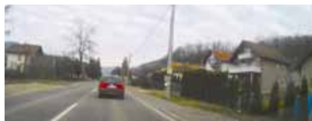
Figure 2. Inadequately protected pillars of electricity distribution and public lighting
