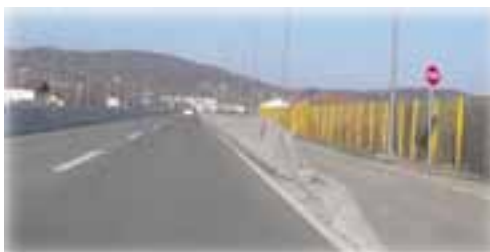
Figure 7. Unprotected new jersey barrier (M16.1)
