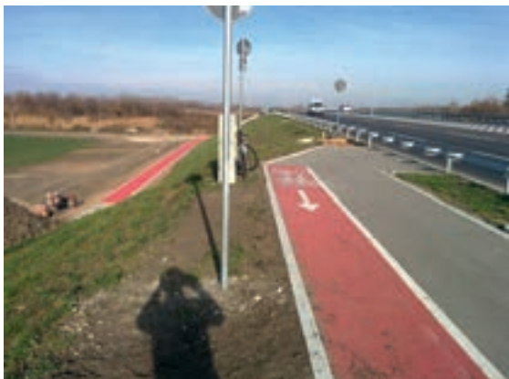
Figure 2. Example of lack of continuity of cycling tracks
