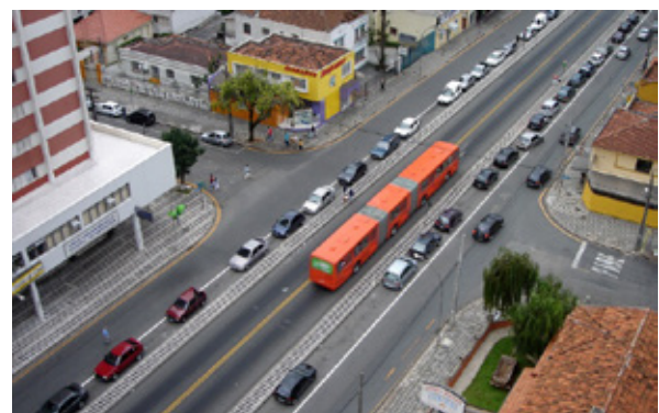
Figure 4. Middle traffic lane intended for BRT vehicles
